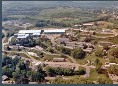
Wolverine supports a 160-acre campus, including more than 100 structures, for NIOSH.
